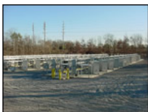
Figure 5: Fuel Cell (PEM) power plant - connected to the grid at LIPA's West Babylon substation
